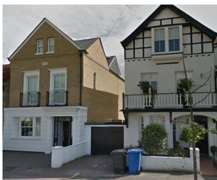
Photo 8 Alma Road. New infill house on the left in keeping with but not the same as its neighbours
