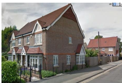
Photo 7 New Houses off Vansittart Road demonstrating local architectural features
